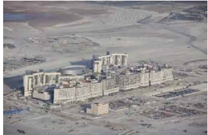
THE NYU ABU DHABI CAMPUS SAADIYAT ISLAND, NEARING COMPLETION
